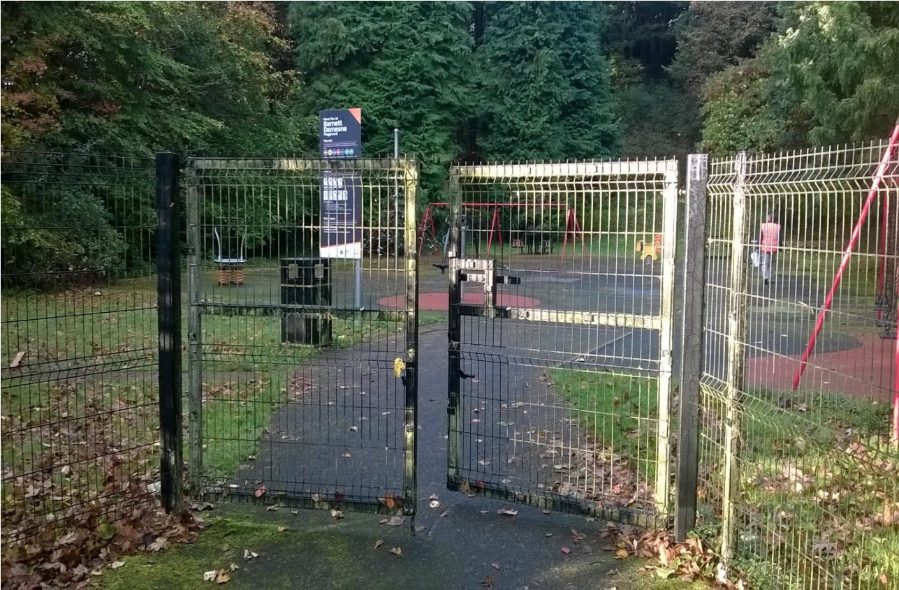
Playground Refurbishment Programme – Shaws Bridge playground (before/ after)
